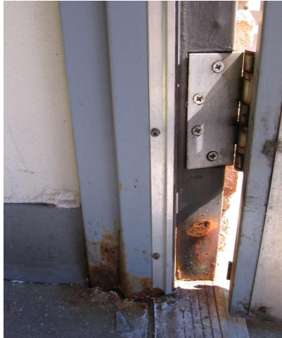
Photo #A25 –rear entrance doors
