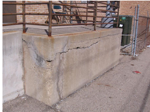
Photo #A8 – south ramp
