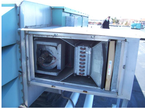
Photo #H7 – Typical pre-heat coil
