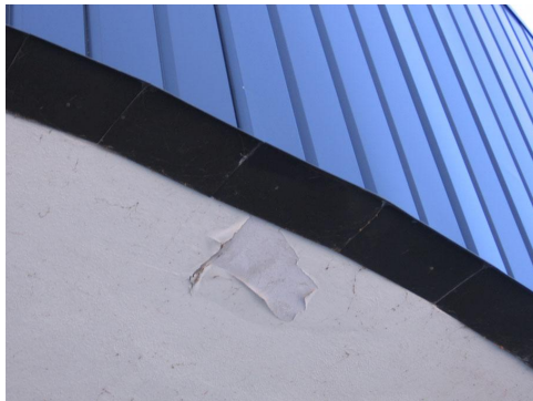
Photo #A21 – exterior canopy soffit
