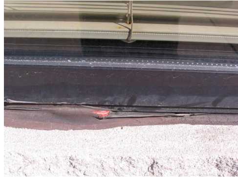
Photo #A20 – window sill detail
