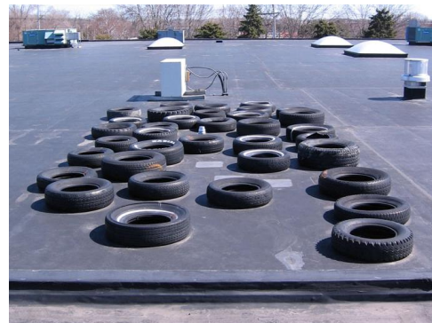
Photo #A28 – non-adhered membrane
