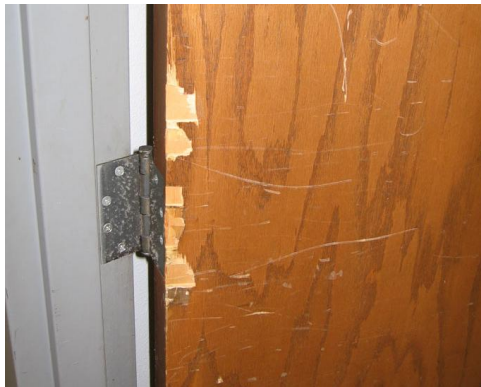
Photo #A33 – interior doors in school
