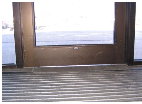
Photo #A24 – 1801 entrance door
