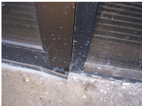
Photo #A23 – 1819 entrance doors
