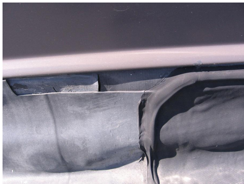
Photo #A27 – perimeter parapet
