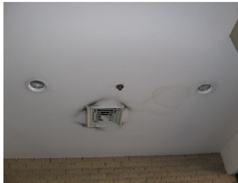
Photo #A34 – Interior ceiling at vestibules
