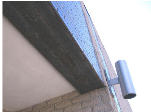
Photo #A22 – steel lintel
