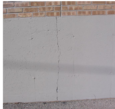
Photo #A40 – foundation wall
