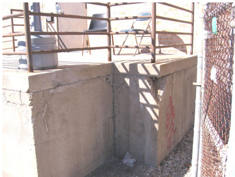
Photo #A9 – south ramp
