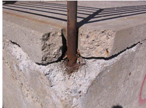
Photo #A14 – east stair / ramp
