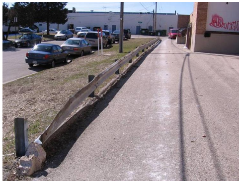
Photo #A15 – south loading area
