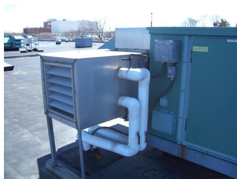
Photo #H6 – Typical pre-heat coil
