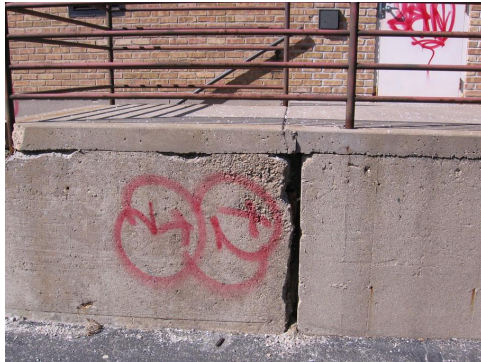
Photo #A13 – east stair / ramp
