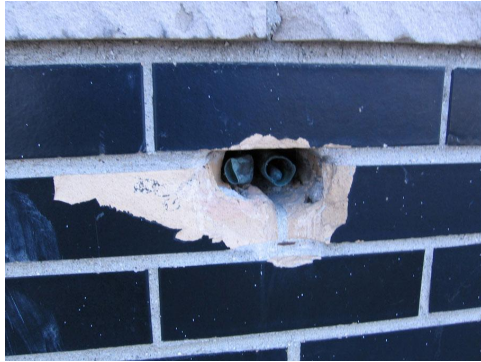
Photo #A19 – north elevation brickwork
