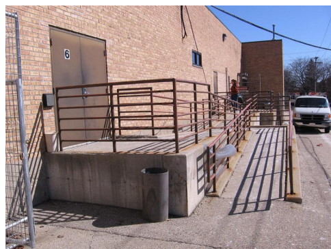
Photo #A6 – south ramp
