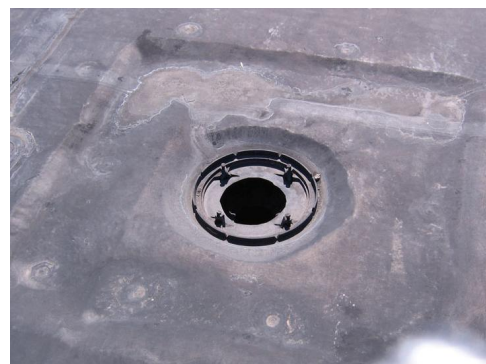
Photo #A30 – roof drain
