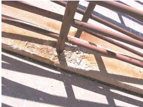
Photo #A7 – typical guardrail condition
