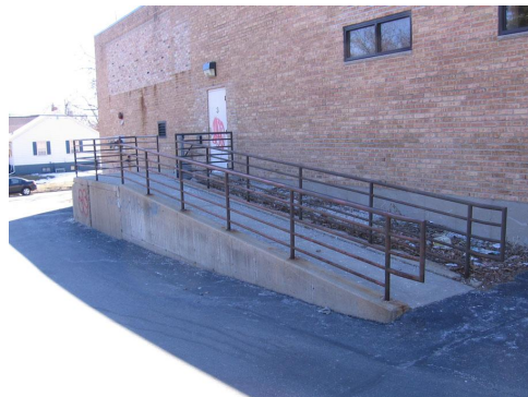
Photo #A10 – east stair / ramp
