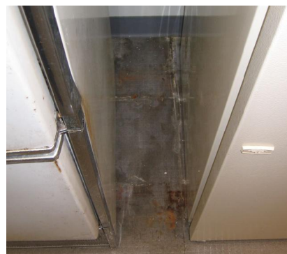
Photo #A36 – break room flooring
