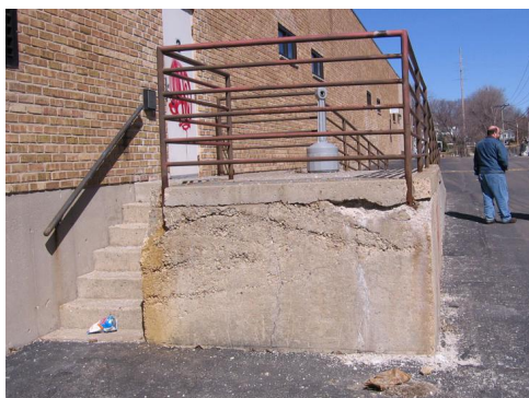
Photo #A11 – east stair / ramp
