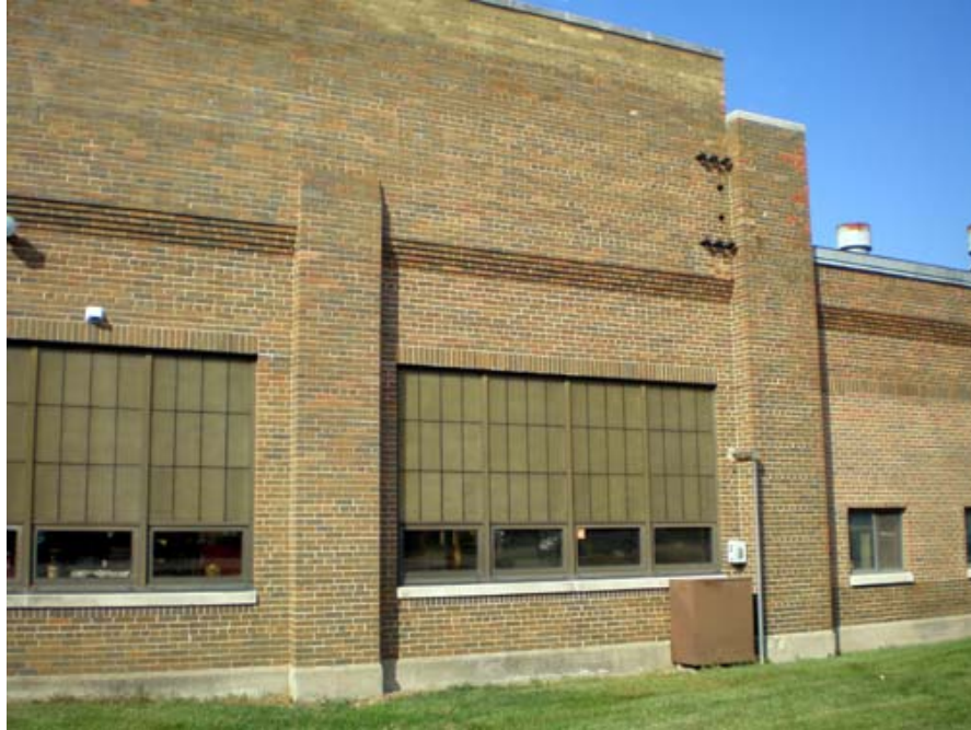
Figure 3 Electrical Service (outside)
