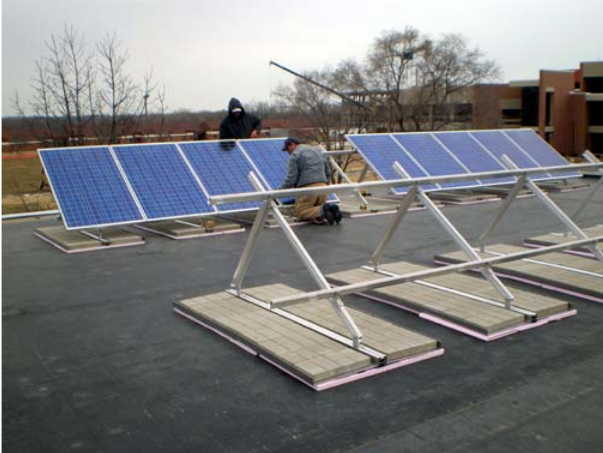
Figure 23 Example Fixed Mounted Pan and Ballast System.
