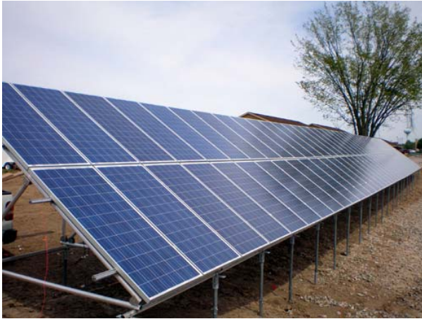
Figure 16 Self Drilling Support Poles.
