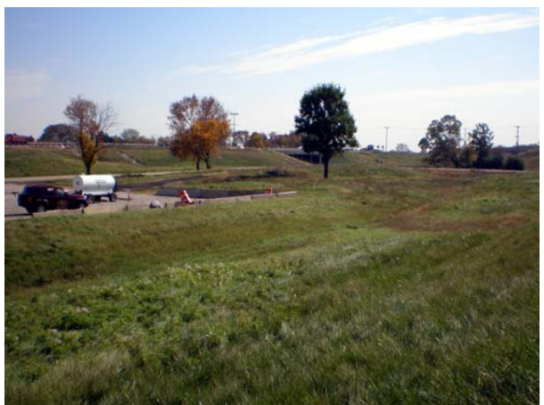
Figure 10 Looking Southeast Highway Embankment.
