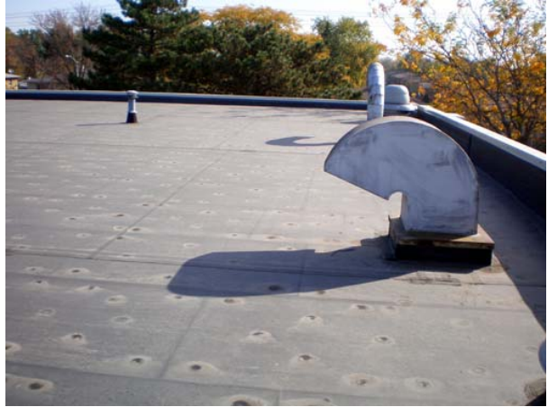
Figure 9 Looking East From SW Corner.
