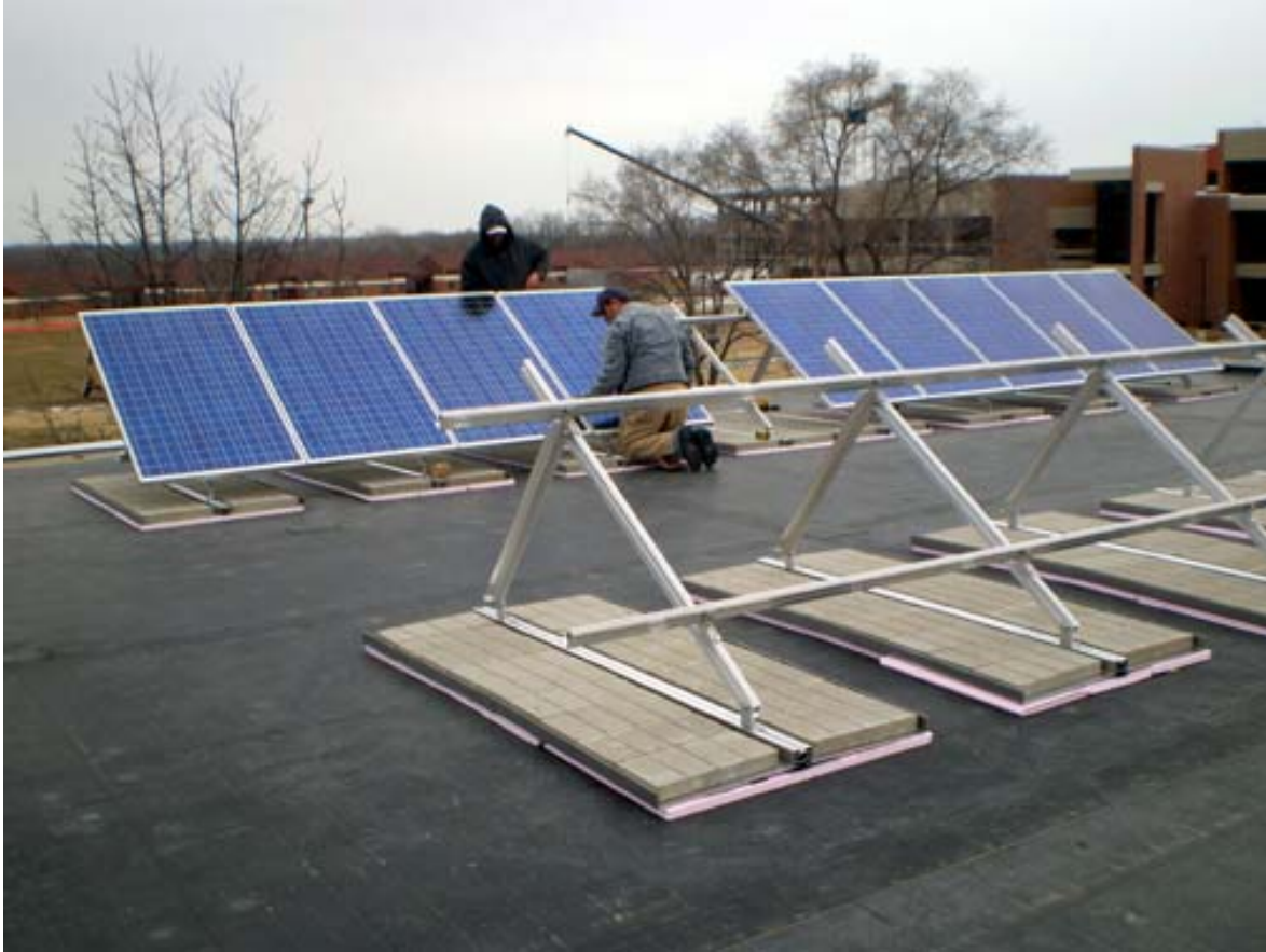
Figure 19 Example Fixed Mounted Pan and Ballast System.
