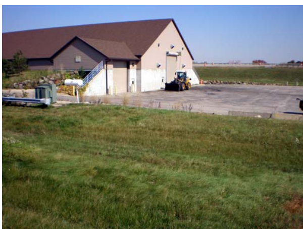
Figure 9 Looking E-SE At Pole Location.
