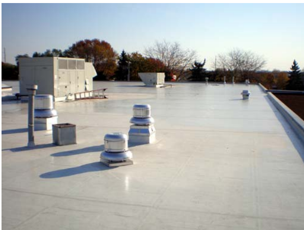
Figure 12 Looking East From SW Corner.
