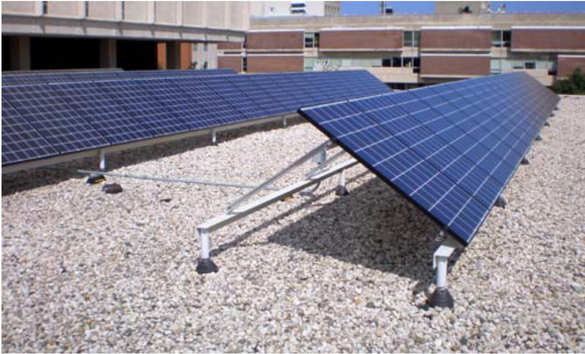
Figure 22 Direct To Roof Mounting System.
