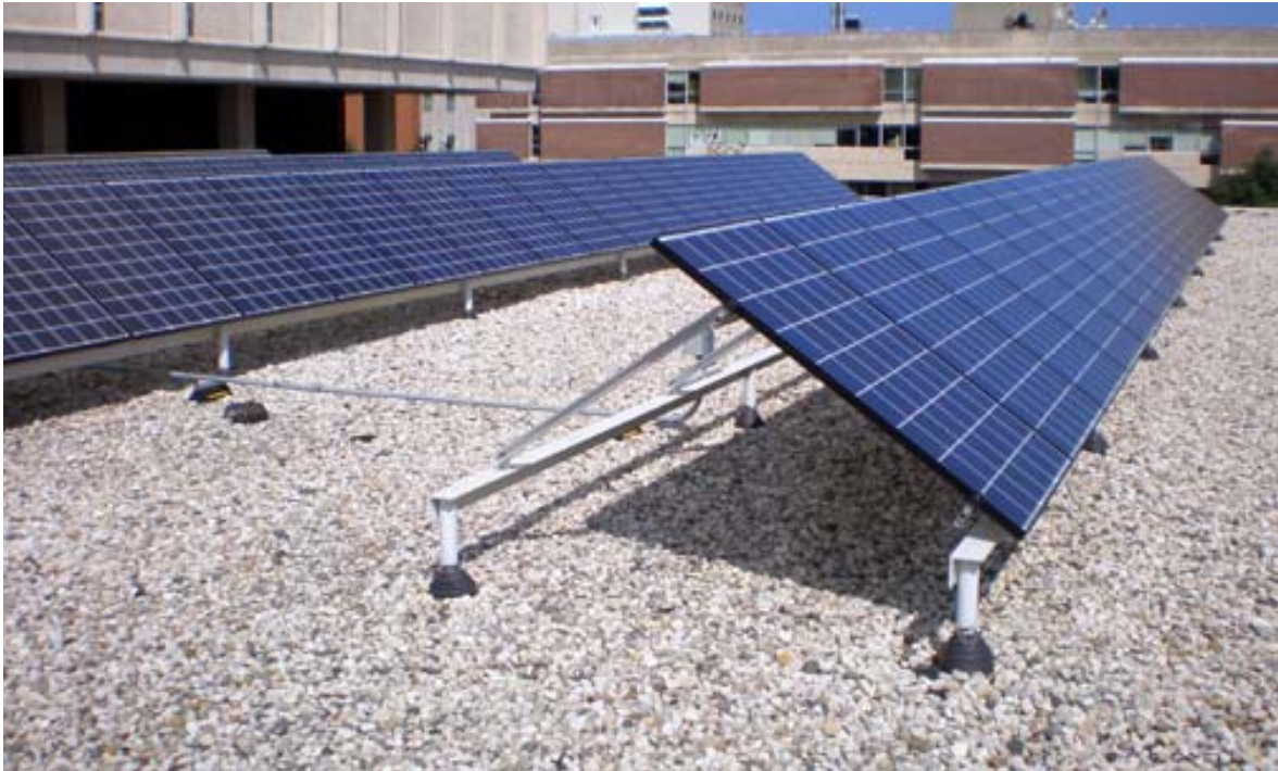
Figure 15 Direct To Roof Mounting System.
