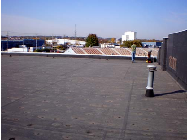
Figure 8 Looking West From NE Corner.
