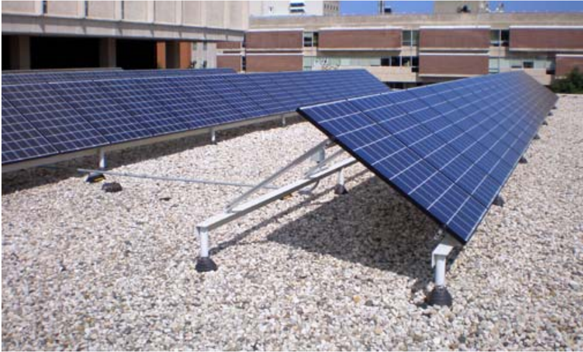
Figure 18 Direct To Roof Mounting System.
