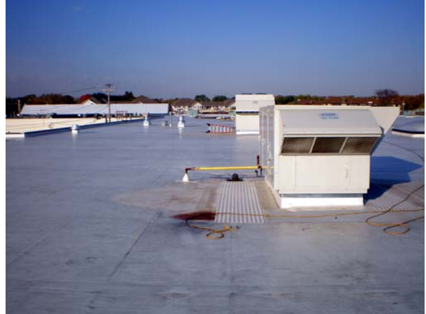
Figure 9 Looking West From NE Corner.
