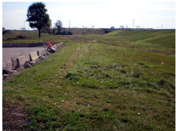
Figure 8 Looking South From Near Pole Location.
