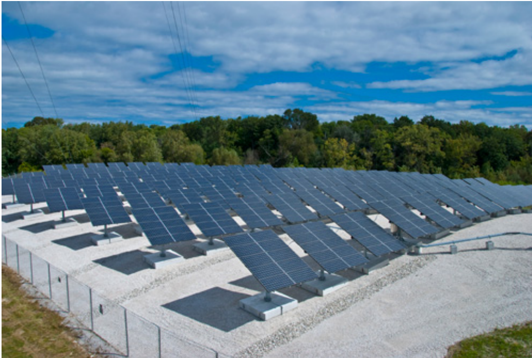
Figure 18 MATC Pole and Slab System. (Photo Courtesy of MATC Web Site)
