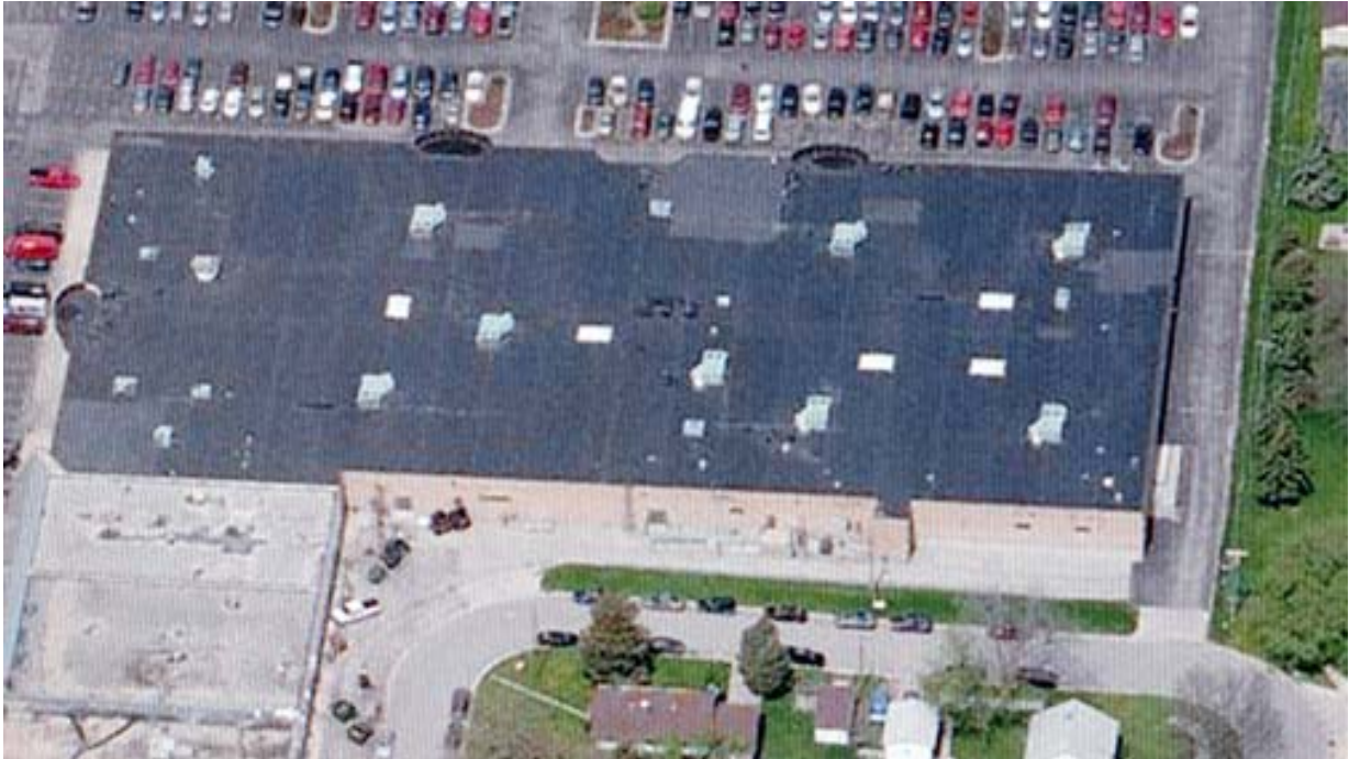
Figure 4 Aerial View Looking North (Photo Does Not Show Recent Changes in HVAC Locations and the Addition of a White Roof Membrane)
