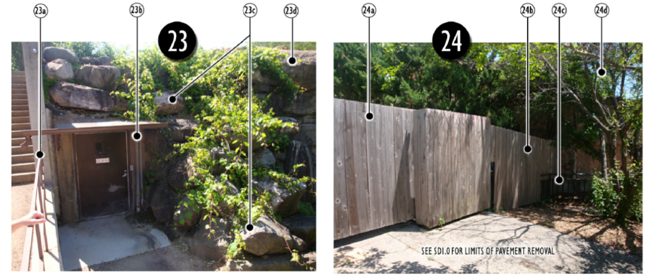
Tunnel/ Service Gate at Admin.
