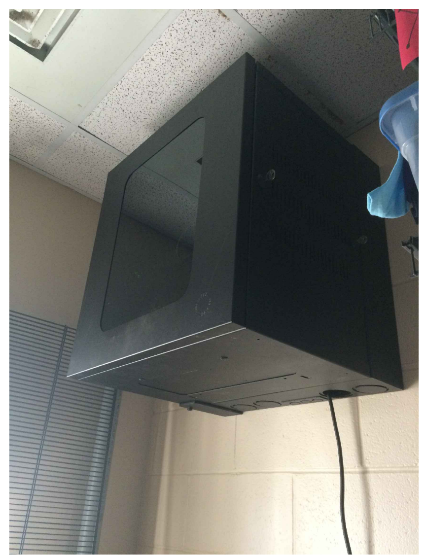
WALL MOUNTED DATA RACK SCALE: NONE
