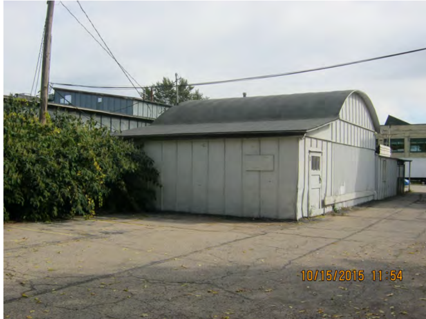
Photo 3: View from the 1316/1318 Washington Avenue subject property parcel from the northwest.
