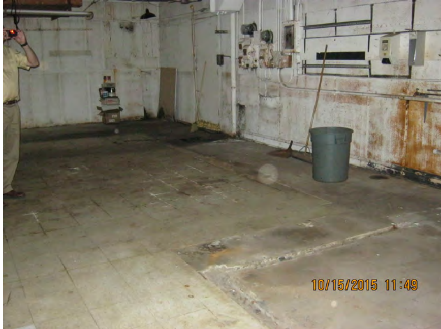
Photo 6: View of the interior of the 1316/1318 Washington Avenue building.
