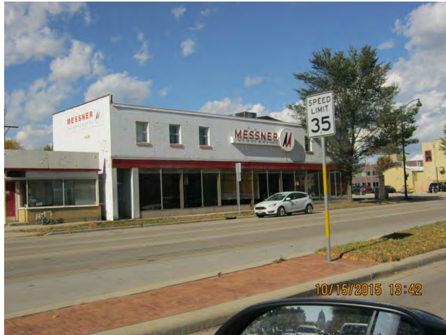
Photo 1: View of the subject property from the south.
