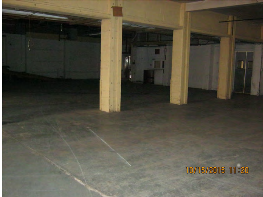
Photo 5: View of the warehouse area in the 1326 Washington Avenue building.
