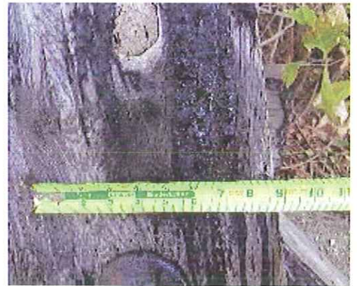
Tar-like material on wood truss:
