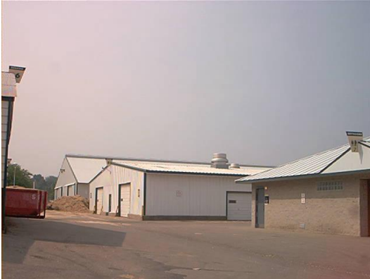
View Looking South West
