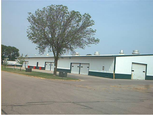
View Looking North West
