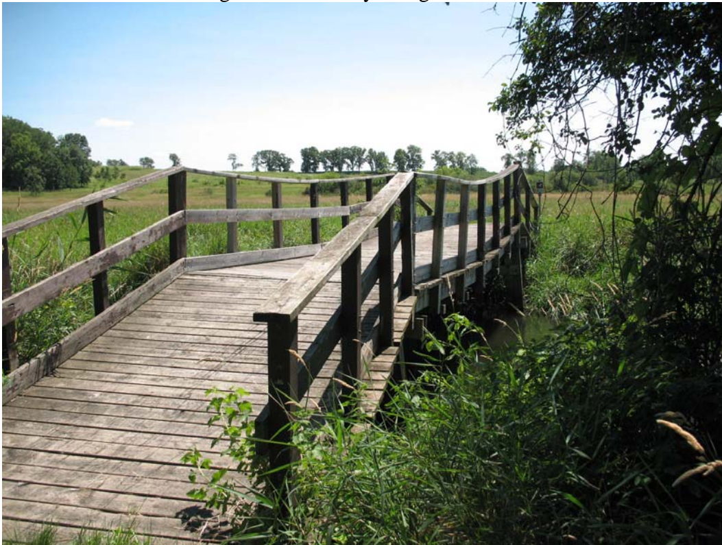
North End of Existing Bridge
