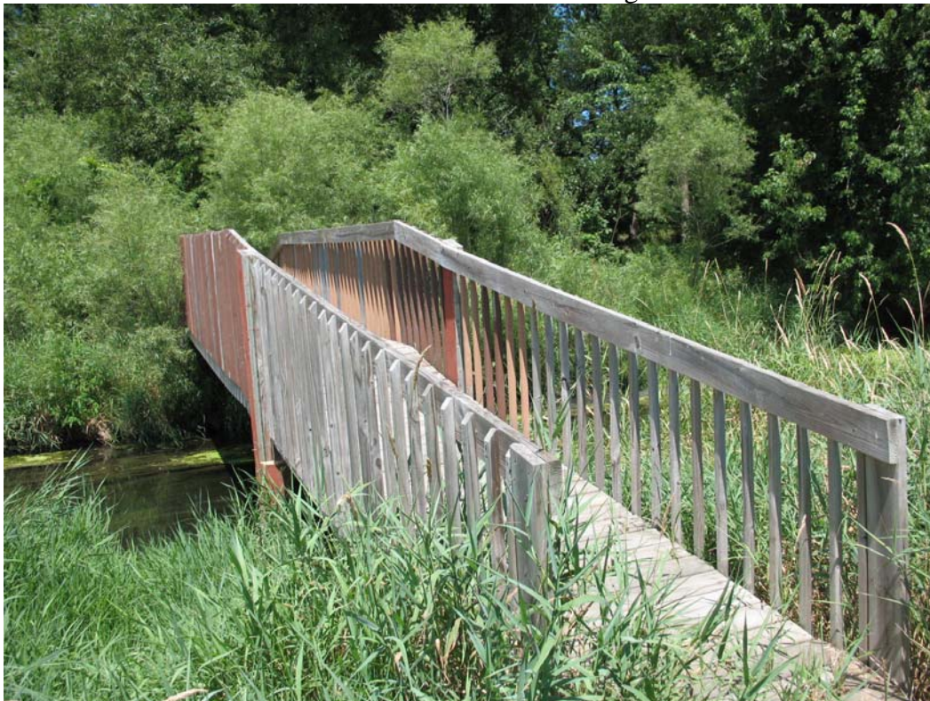
South End of Existing Pedestrian Bridge
