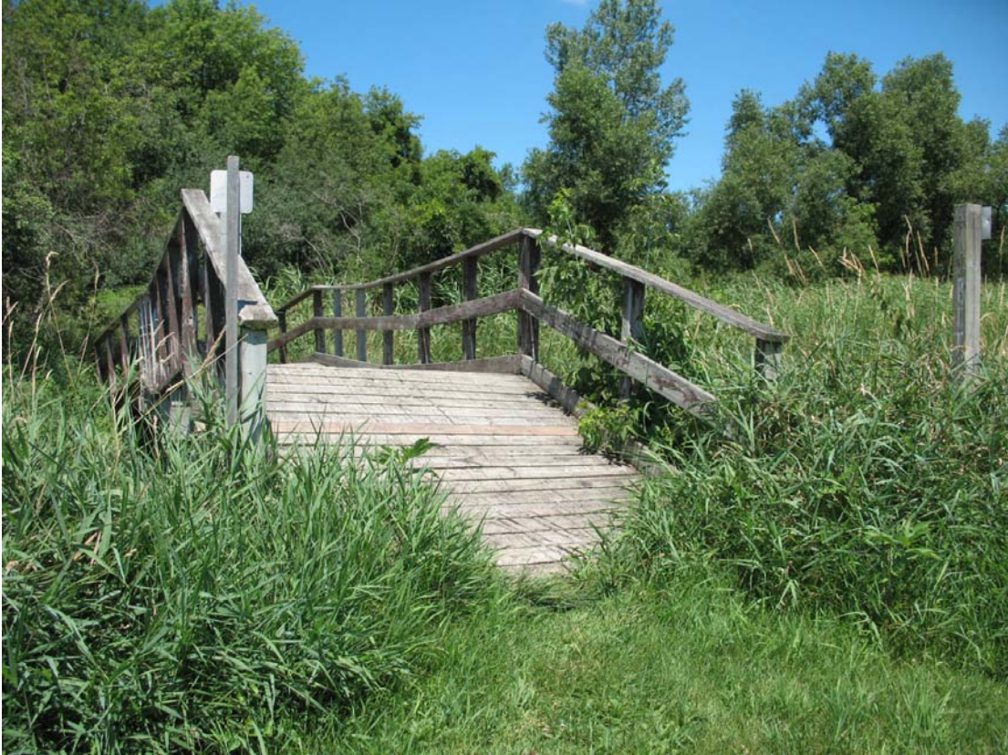
South End of Existing Bridge
