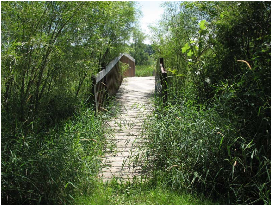
North End of Pedestrian Bridge
