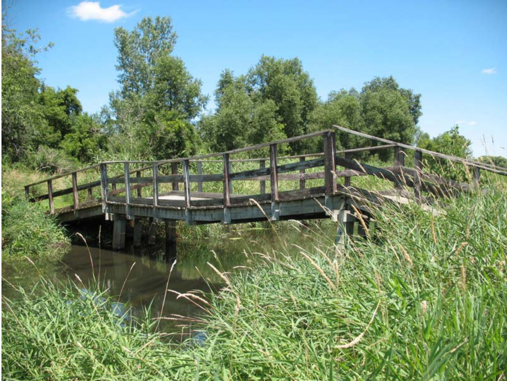
Existing Rustic Parkway Bridge to be removed
