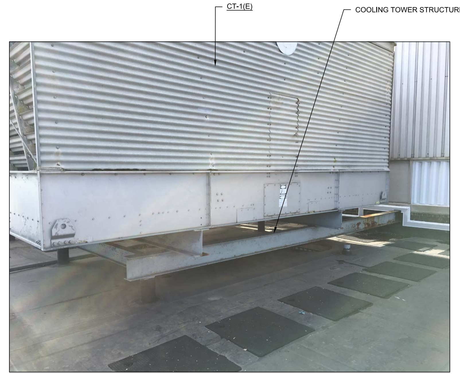
4 PHOTO - WEST SIDE OF COOLING TOWER ME101 SCALE: N.T.S.
