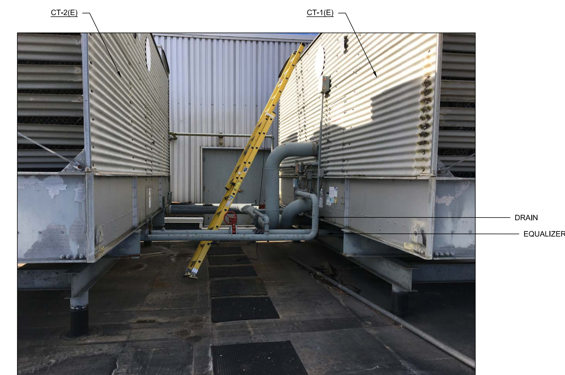
3 PHOTO - LOOKING BETWEEN COOLING TOWERS ME101 SCALE: N.T.S.
