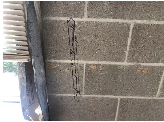
Rebar Scan #2- Rebar marked in black sharpie.
