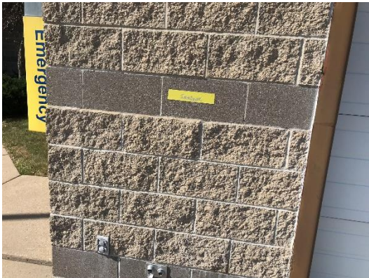
Area #6 Inconclusive scan area.
