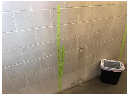
Area #2- Field Marks- Tape with marker showing center of vertical bars.
