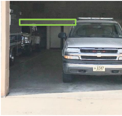
Bond Beam Scan Location (Green Box)
