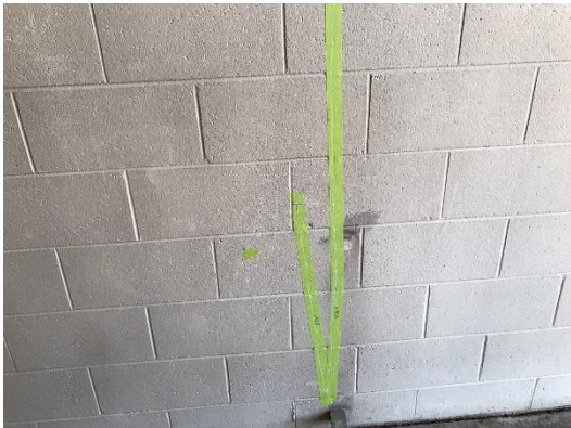
Area #1- Field Marks- Tape with marker showing center of vertical bars.
