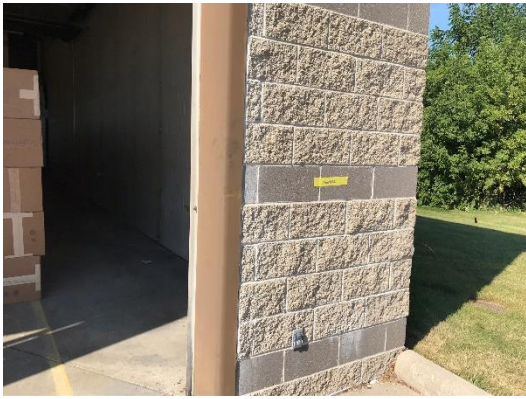
Area #7- Inconclusive scan area.
