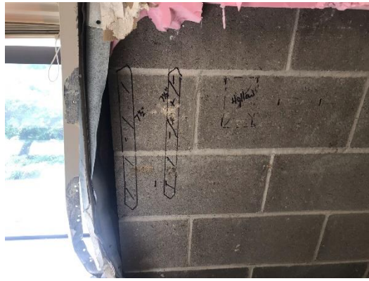
Rebar Scan #3- Rebar marked in black sharpie.
