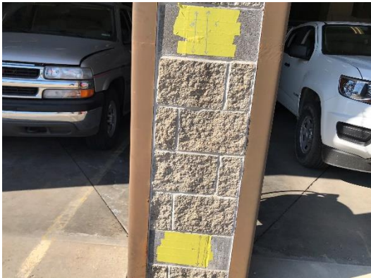
Area #5 Field Marks- Tape with marker showing center of vertical bars.
