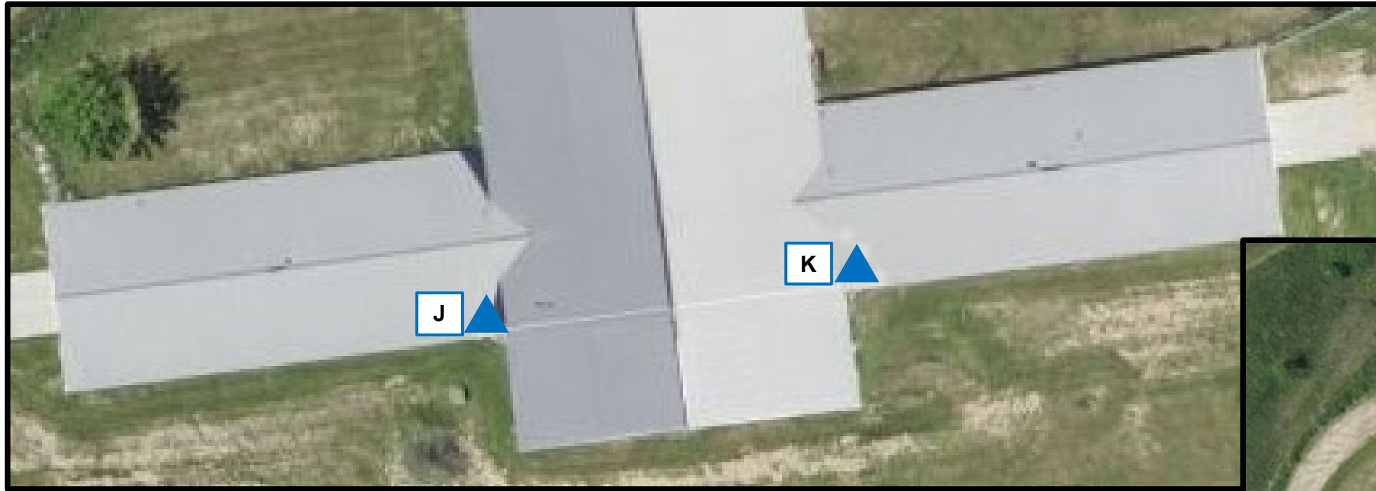
Alternate Bid 1: roof panel repairs at locations J & K
