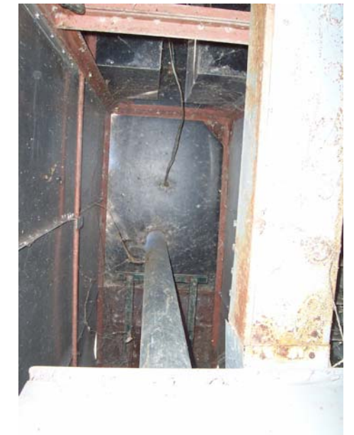
LOOKING UP INTO STRUCTURE
