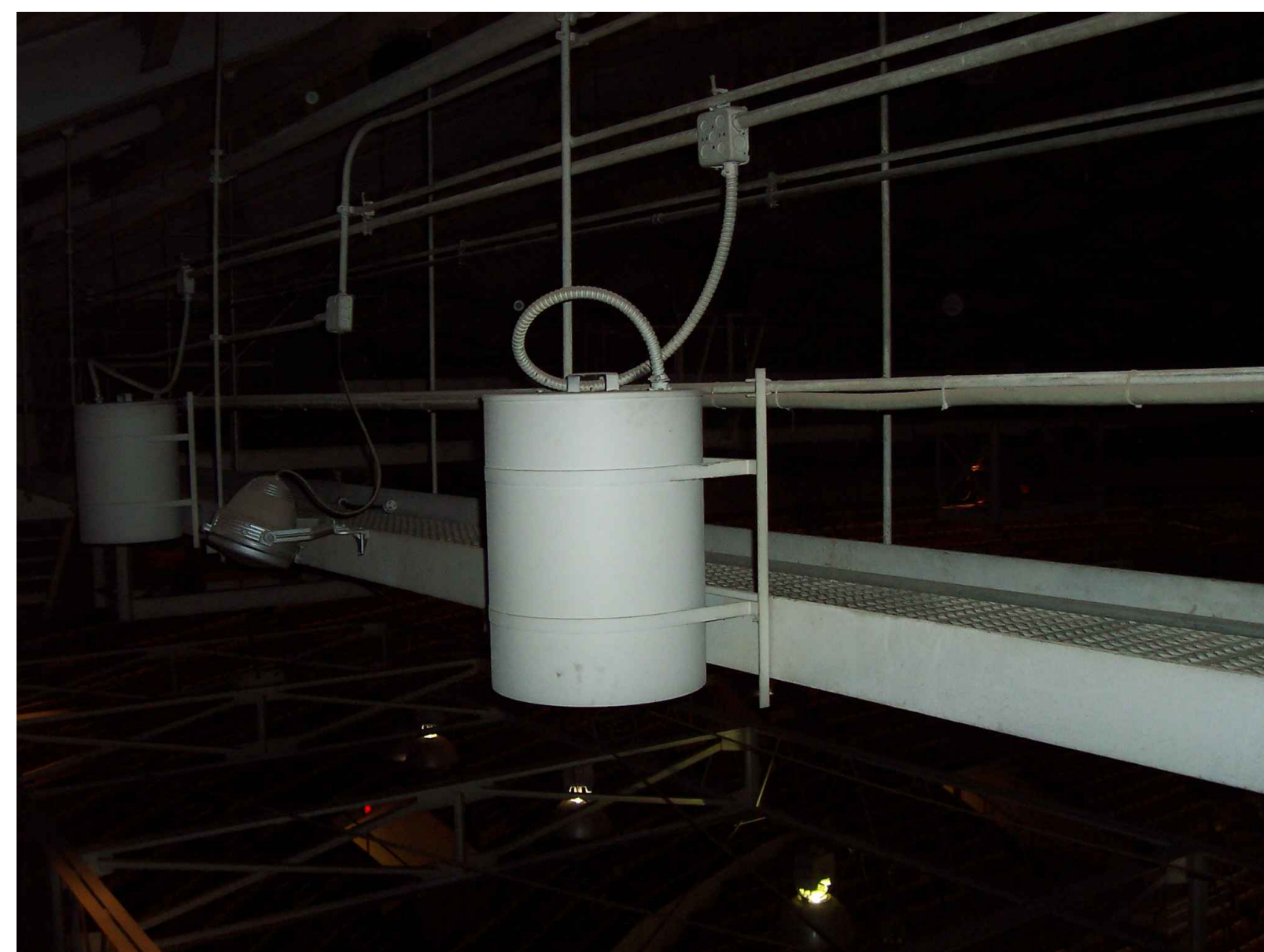
LIGHTS AT CATWALK
