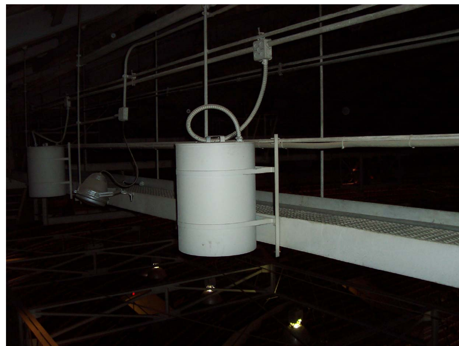
LIGHTS AT CATWALK
