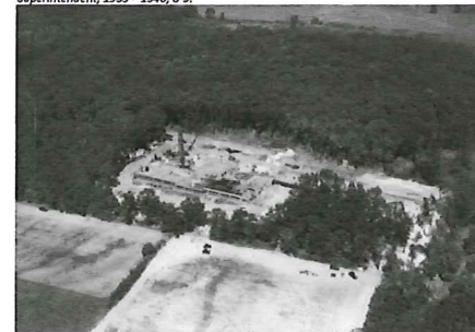
Lake View Sanatorium under construction, 1929 (source: Wisconsin State Historical Society Archives, 35103, by Arthur M. Vinje).
