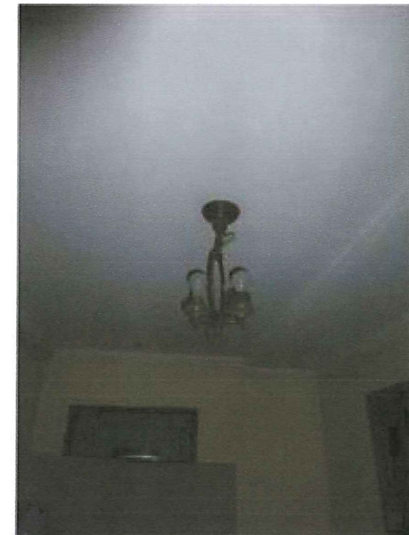
Image 10 Original light fixture, main entry, first floor
