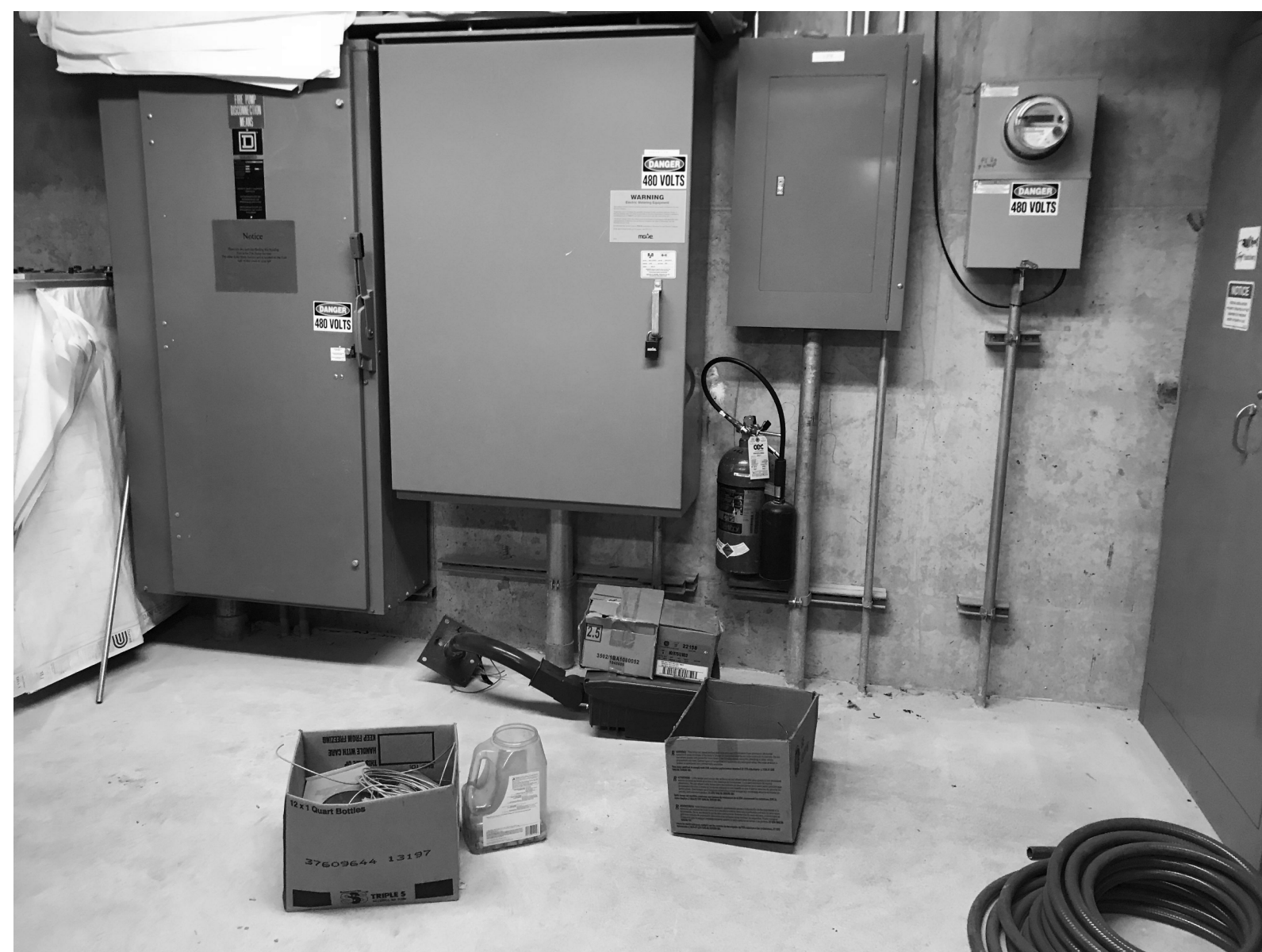
4 FIRE PUMP DISCONNECT - ELECTRICAL ROOM SOUTH WALL NO SCALE
